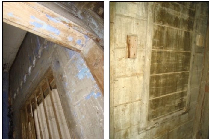
Figure 13. Traces of the first original building period: iron-barred guillotine window and wooden covered guillotine window (Tanrıverdi, 2011)
