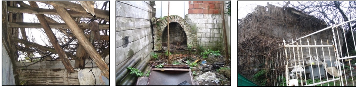
Figure 16. Woden roof and biological deterioration (Tanriverdi, 2011)
