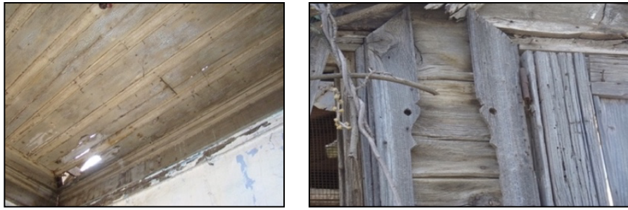
Figure 14. Wooden lathed ceiling of room Z-02 and the wooden decorations around the guillotine window (Tanriverdi, 2011)
