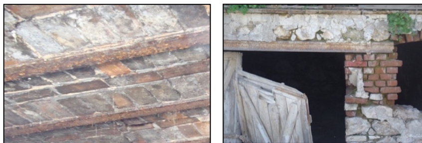
Figure 15. Deterioration of the metallic elements (Tanriverdi, 2011)
