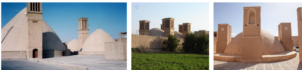
Figure 5: Several views of Ab-Anbars with badgirs towers (wind-catchers)
